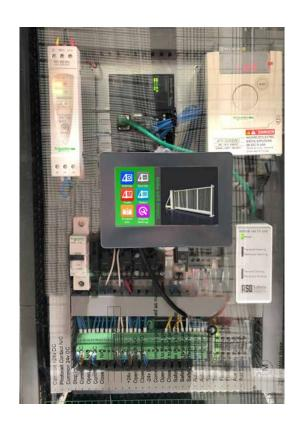
Our new optional touch screen display extends the capabilities of our control system and allows you to set up and configure the system in a matter of minutes.
